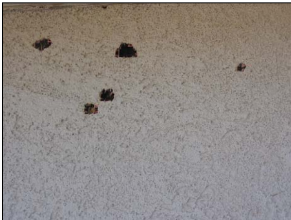
Holes in the stucco material at the north and west sides of the addition.
