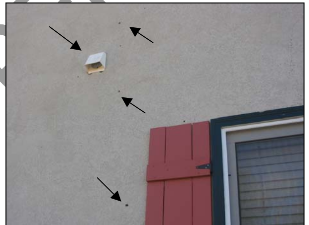
Holes in the stucco material at the north and west sides of the addition.
