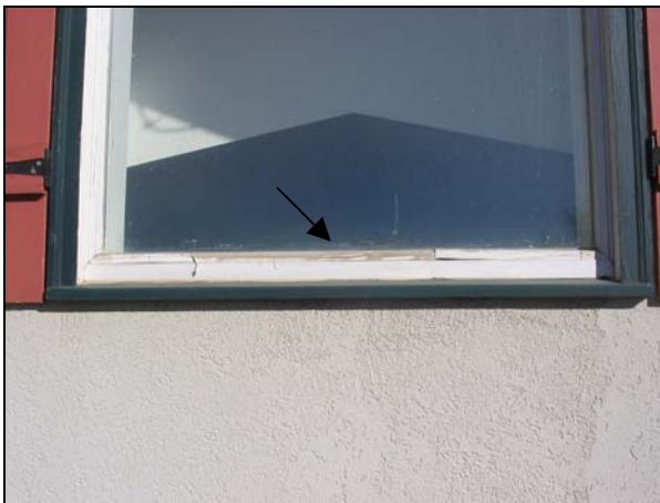
Window trim paint is peeling at various locations.
