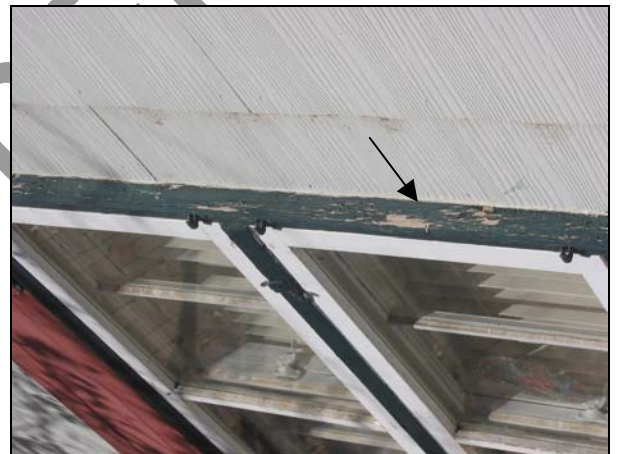
Window trim paint is peeling at various locations.
