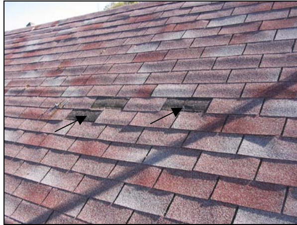
West slope of the detached garage.
